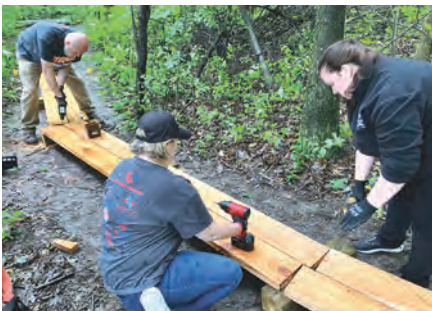
Volunteers from Meijer Scio Twp #173 install a boardwalk at Johnson Preserve.
