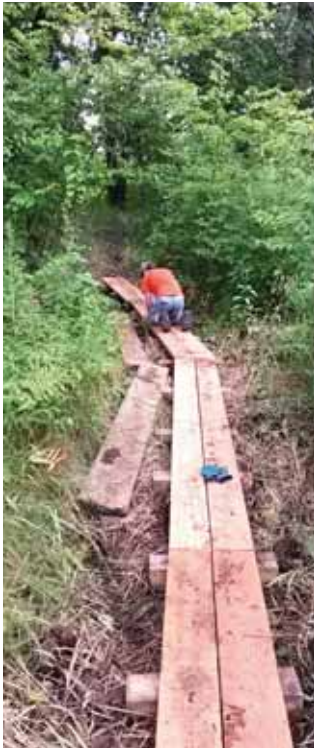
Boardwalk Replacement at Reichert Preserve
