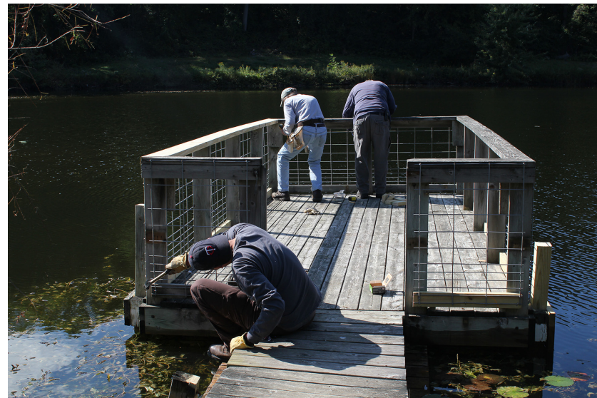
Figure 10 Floating dock repair in the fall of 2014
