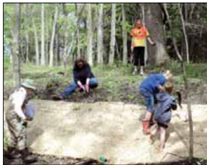
Volunteers plant into erosion blanket on the banks at Beckwith.
